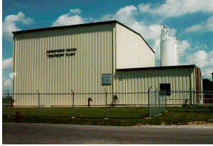
WTP Operations Building.
