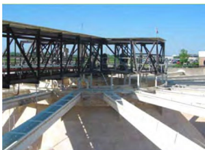
The PAWP, which originally went into service in 1984, draws water from wells and provides 16 percent of the water in the service area. For the recent $65M upgrade, we provided extensive construction sequencing of many connection points to existing facilities with no disruptions to water production during construction and startup.
