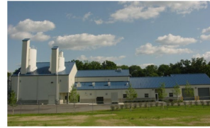
Versailles new 1.5 MGD lime-soda-ash softening WTP.
