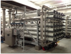
Membrane Softening Process.
